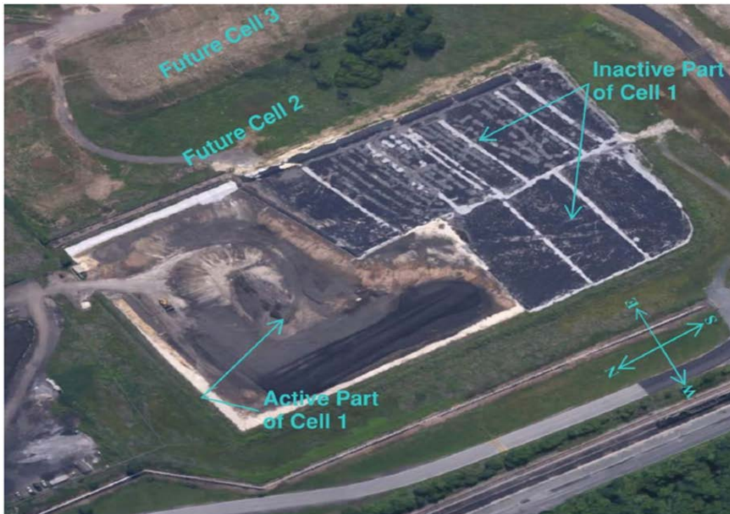
Photo 1 - Aerial view of Brunner Island Ash Area No. 8. The active part of Cell 1 is seen to the left (north). The right (southern) part of Cell 1 has had the liner system installed, but has not been filled. Temporary plastic tarps can be seen covering the liner system over the inactive part of Cell 1. Construction of Cells 2 and 3 has not yet started.
