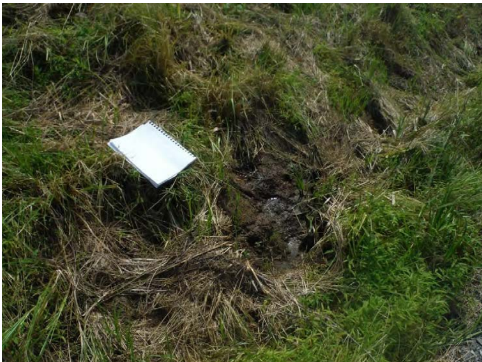
Figure 11: Standing Water at the Toe of the Slope at the North End of the West Embankment
