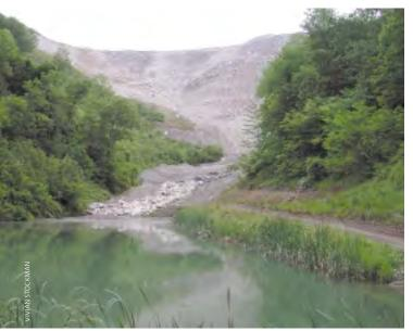
Valley fills are created when waste rock is dumped from the mining area into nearby stream valley – sometimes over two miles long. This is a picture of a small valley fill in its early stages. The pond at the toe of the fill is meant to prevent sediment from entering the rest of the stream. Fills under construction often contribute to downstream flooding when rains rush off the denuded mining area above overwhelming the ponds and causing them to break or overflow.
